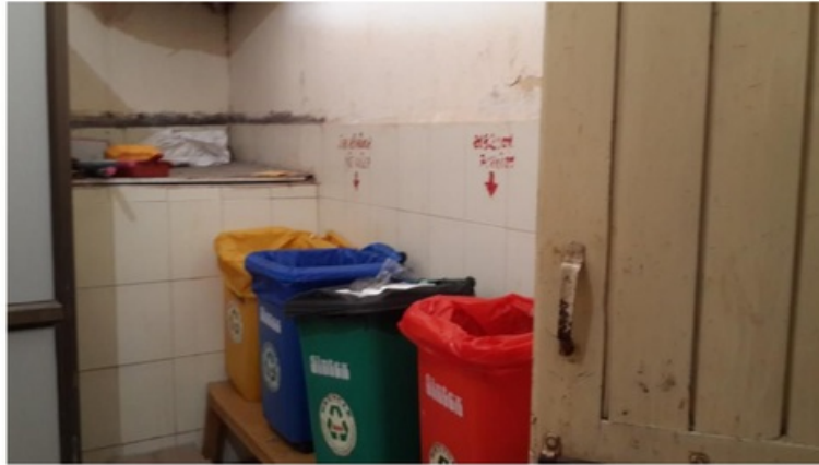
Segregation of Waste
